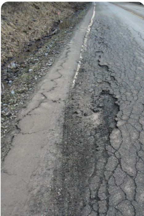
Road damage from heavy trucks, West Virginia
