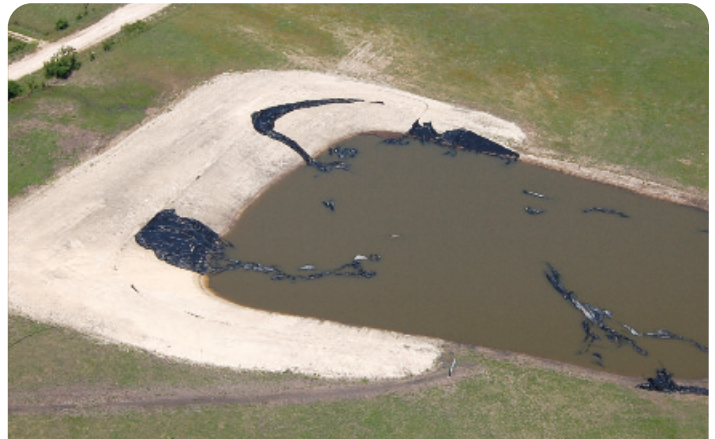
CREDIT: EARTHWORKS Action Damaged lined waste pit
